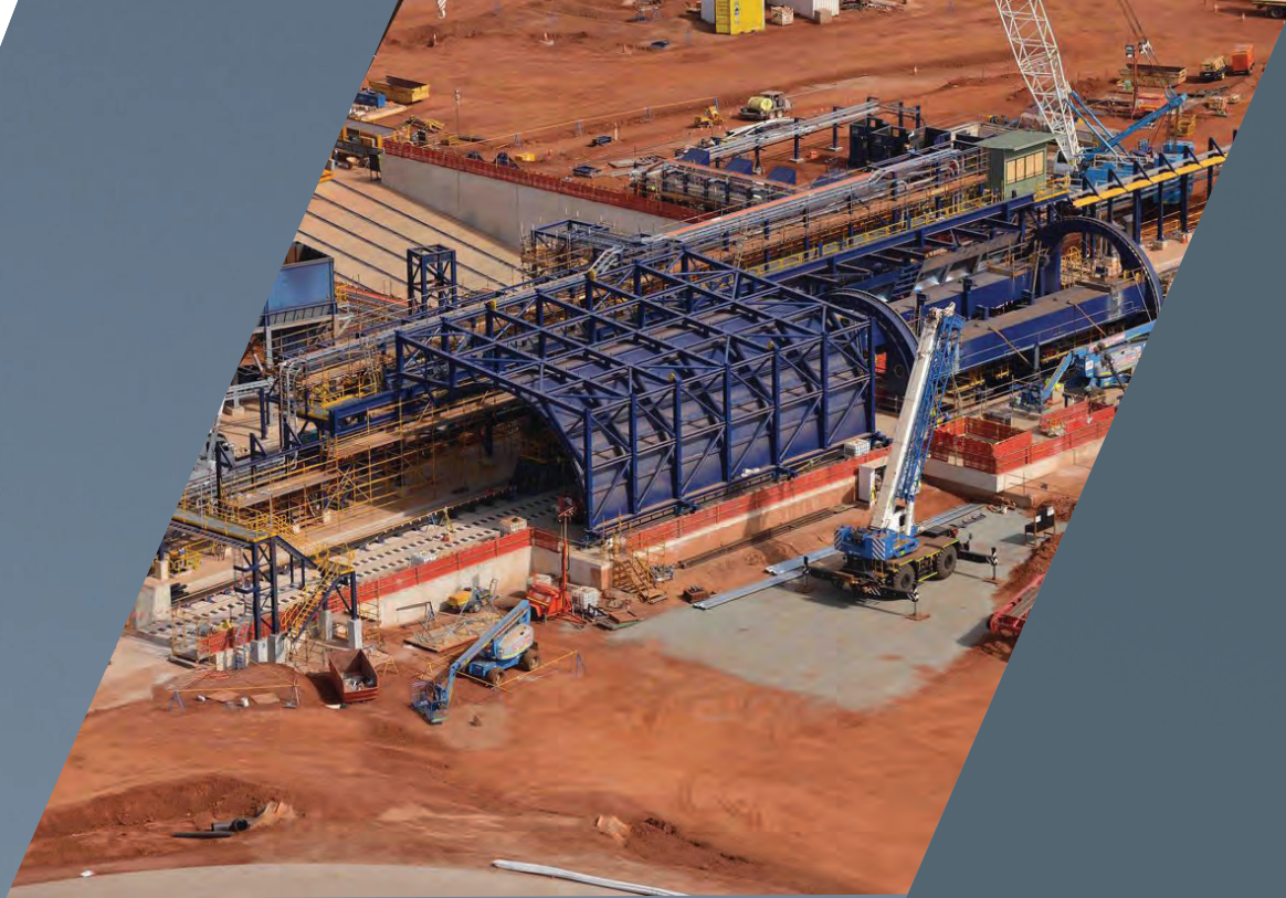
PHOTO: This rail car dumper was installed by Civmec crews on the Roy Hill Project in WA's North West.
