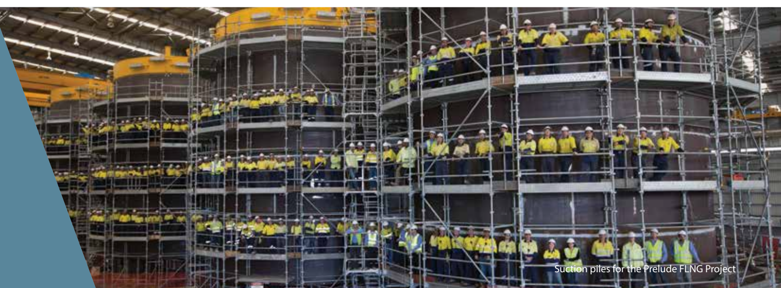
Assembly of spools for the Prelude FLNG Project
