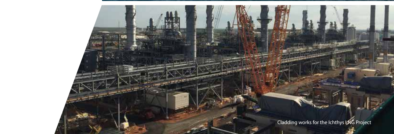
Load out of jumper spools for the Wheatstone LNG Project
