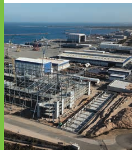
New shipbuilding and maintenance facility currently under construction, Henderson, Western Australia
