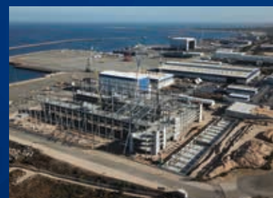
New shipbuilding and maintenance facility currently under construction, Henderson, Western Australia
