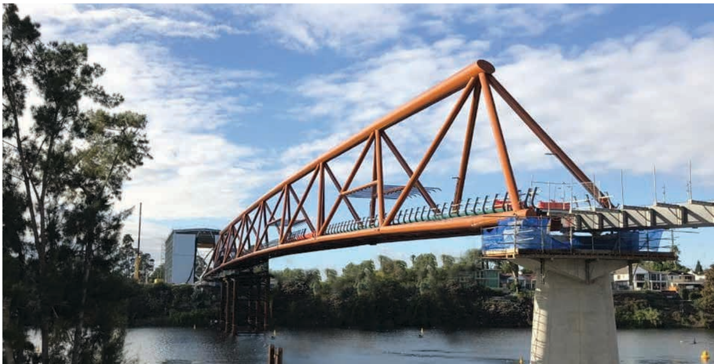
Nepean River Bridge, Penrith, New South Wales
