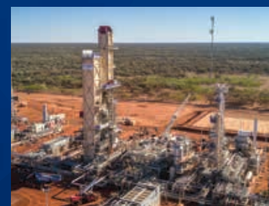
Phillip Creek Gas Treatment & Compressor Station (Northern Gas Pipeline), Tennant Creek, Northern Territory
