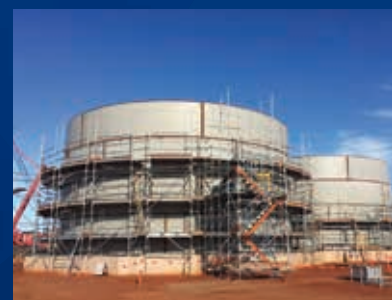
Gruyere Golds Project, Goldfields, Western Australia
