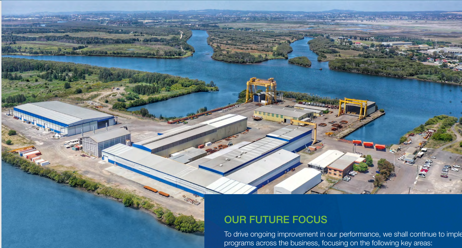
Aerial view of east coast facility, Newcastle, New South Wales
