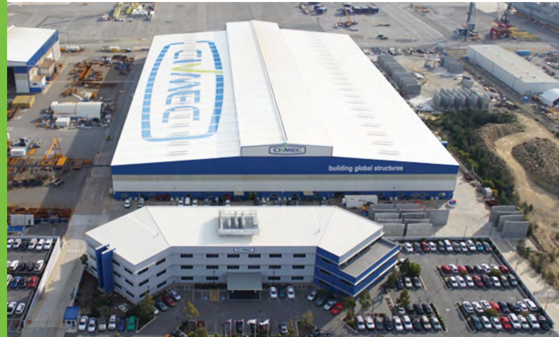
29,300m 2 heavy engineering workshop, Henderson, Western Australia
