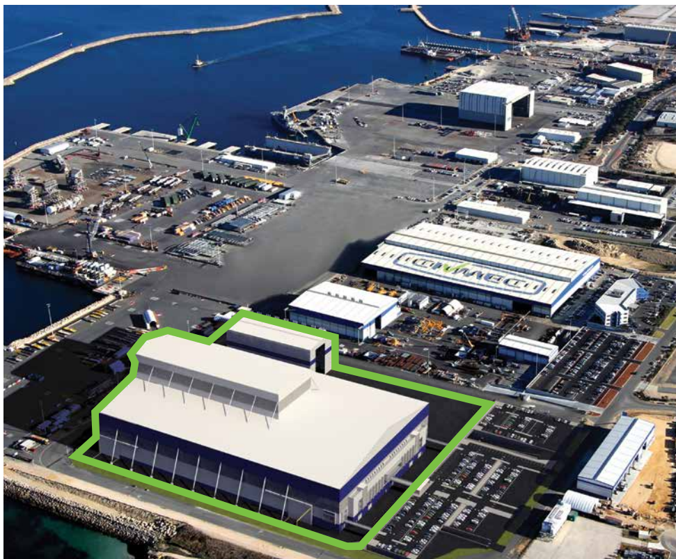
Henderson facility – current and future (showing development in green outline for completion in Q4 2019)
